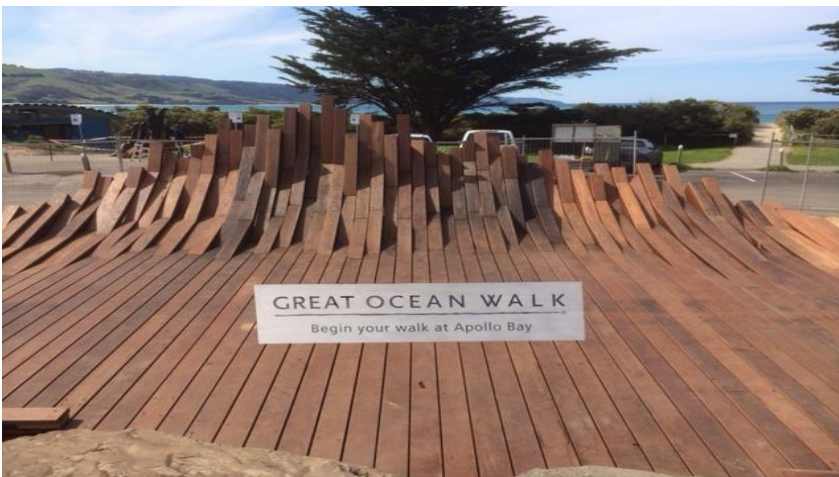
COMPLETED GREY IRONBARK DECK FEATURE
